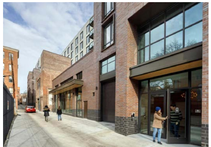
Entrances activate the alley between W and V streets on the rear of Collection 14 with access to retail, leasable office space, and event space. Source: perkinseastman.com.
