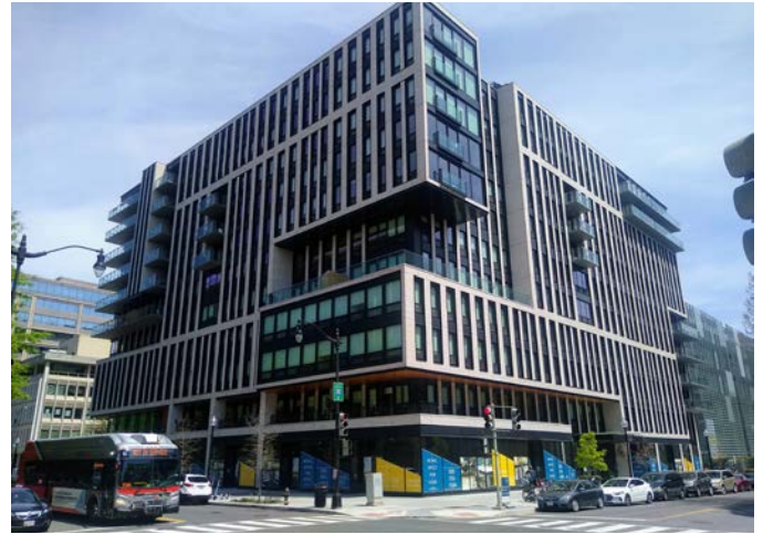
The building massing of 555 E Street SW is articulated with both horizontal and vertical breaks, accommodating balconies and terraces at various levels.
