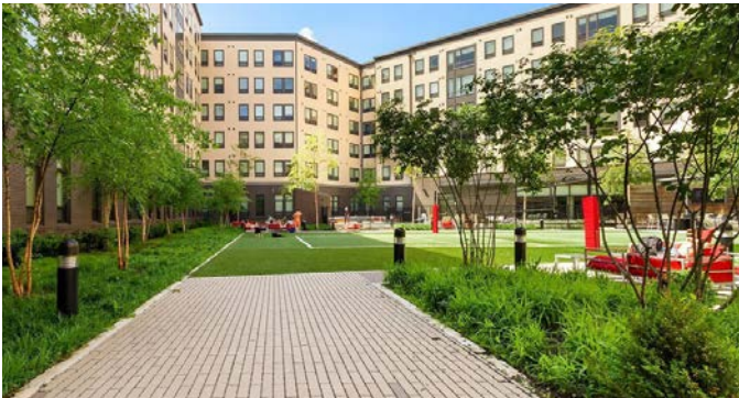
Open spaces on the proposed bus garage could include pathways, seating areas, play structures, vegetation, and gardens, like at Terrapin Row in College Park, MD. Source: parkerrodriguez.com .
