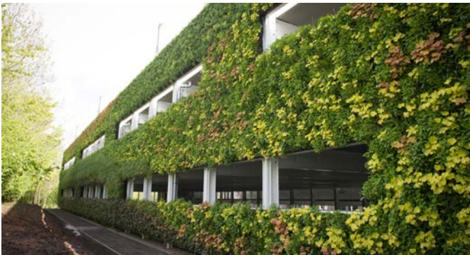
A living green wall could be employed on the southern and 45th Street façades of the proposed garage, like this one in Warwick, UK. Source: archello.com .
