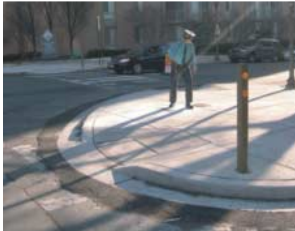
Our new intersection bumpout at South Park/Hills Plaza improved pedestrian safety.
